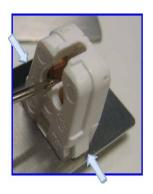
Disconnect the wires of the neon tube holder to be replaced, by using a suitable tool.
