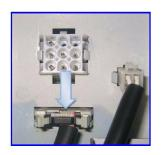
7.2 Check if the connector inside the extractable unit column is connected properly.
