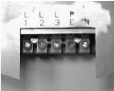
electrical connection ESW 308.6
