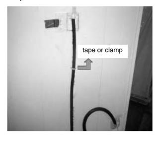
Insert the black drain tube (electrical tube) into the white drain spout and fasten it to the back wall using tape or a plastic clamp.
