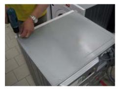
2. Remove the screws from the top cross bar.
