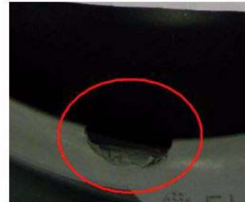
c) Piece torn out of the seal
